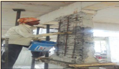
Strengthening of Column
