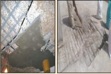
Repairs with PMR Mortar
