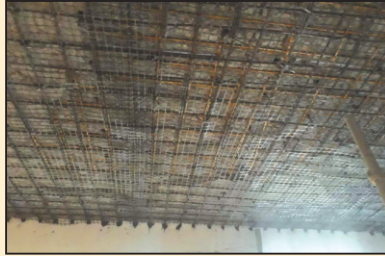
Strengthening of Slab
