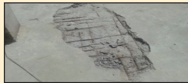
Terrace Flooring Patch Works
