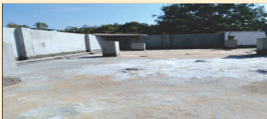
Terrace Flooring New
