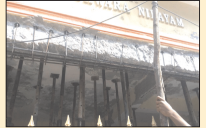
Strengthening of Beam
