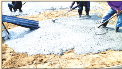
Ground Level Flooring
