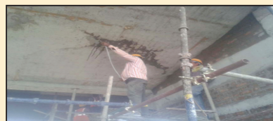
Pressure Grouting
